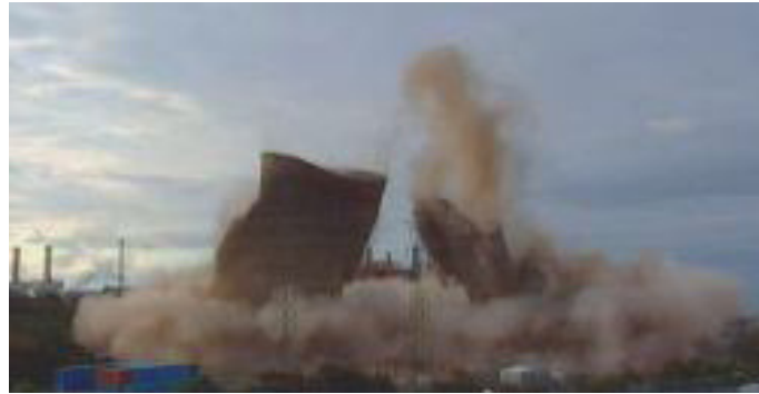
(b) Controlled collapse of each tower.
