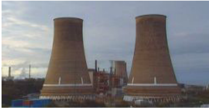
(a) Explosive charges are placed under the towers.
