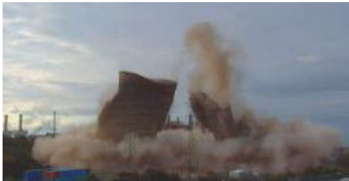
(b) Controlled collapse of each tower.
